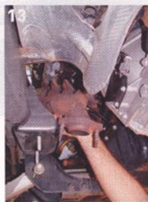
Both exhaust manifolds were then unbolted and removed.
